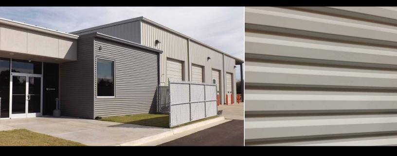
MasterLine 16® is a concealed fastener metal wall panel that provides an interesting shadow line, enhancing the aesthetics of the panel. While primarily designed for horizontal applications, it can also be installed vertically to give a distinguished architectural design. The panels provide 16" coverage and are available with factory applied mastic in the side laps. Panels may be attached to metal studs, with or without sheathing, as well as to subgirts.
