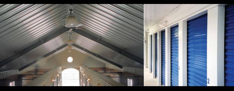
The PBR panel is commonly used for a wide variety of architectural, agricultural, commercial and industrial applications. PBR is a structural panel and an exposed fastener panel that can be used for both roof and wall applications. The minimum roof slope for PBR is 1/2:12.
