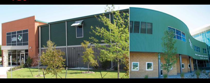
The PBU panel is an exposed fastener system that can be used for both roof and wall applications. PBU can be installed directly over purlins or joists. PBU offers the versatility of being used in both vertical and horizontal applications to give designers a contemporary appearance for their building project. PBU is recommended for 1:12 or greater roof slopes.
