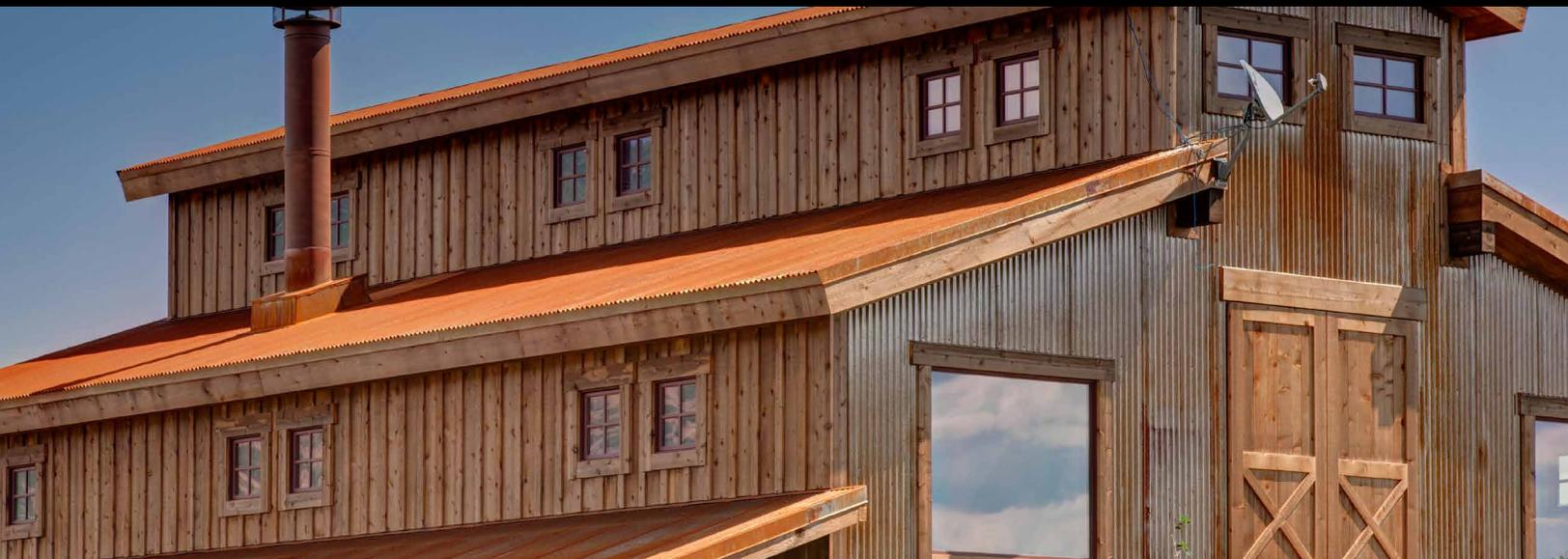
Metallic's Rustic C Panel is the ultimate roofing panel for innovative builders who choose the beautifully weathered look of rusted steel. Designed to weather and naturally oxidize, Rustic C Panels provide a picturesque western look. The Rustic C Panel is recommended for installation in arid and semi-arid climates.
