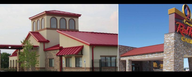
The Ultra-Dek® roof panel is a snap-together, trapezoidal leg standing seam roof system. Ultra-Dek® panels are available in 12-inch, 18-inch and 24-inch widths. Ultra-Dek® requires a minimum slope of 1/4:12 and is ideal for industrial, commercial and architectural applications. Ultra-Dek® can be erected on various types of construction.
