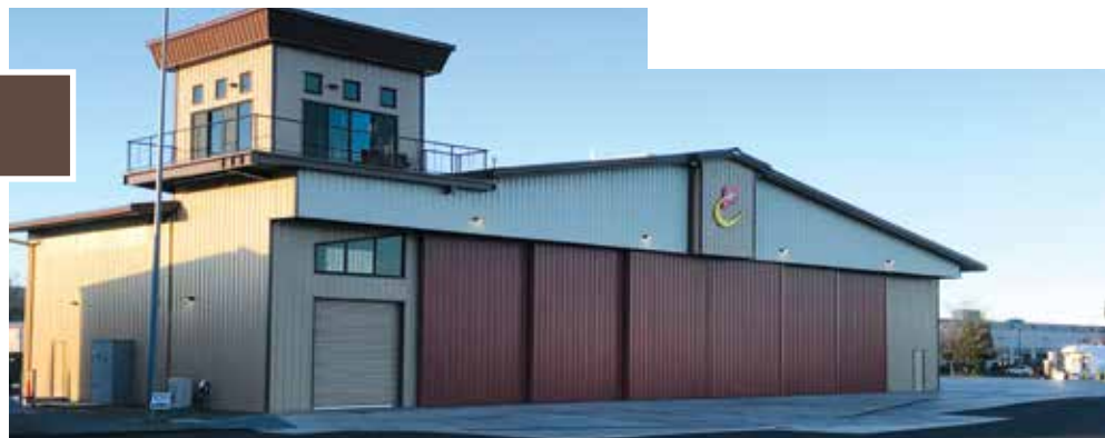
PROJECT: FLYERS ENERGY HANGAR
