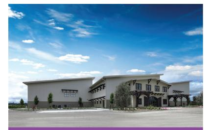
The winery is a mixed-use facility that includes office space, a tasting room, a crush pad area, a fermentation room and spacious barrel storage. This project consists of a custom-engineered metal building system and IMPs.
